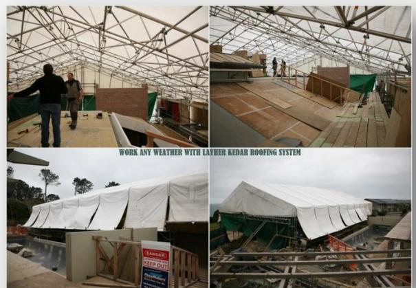
Keder Roof with Scrim (green netting) around the building to protect from the weather and keep the dust and debris on the construction site
